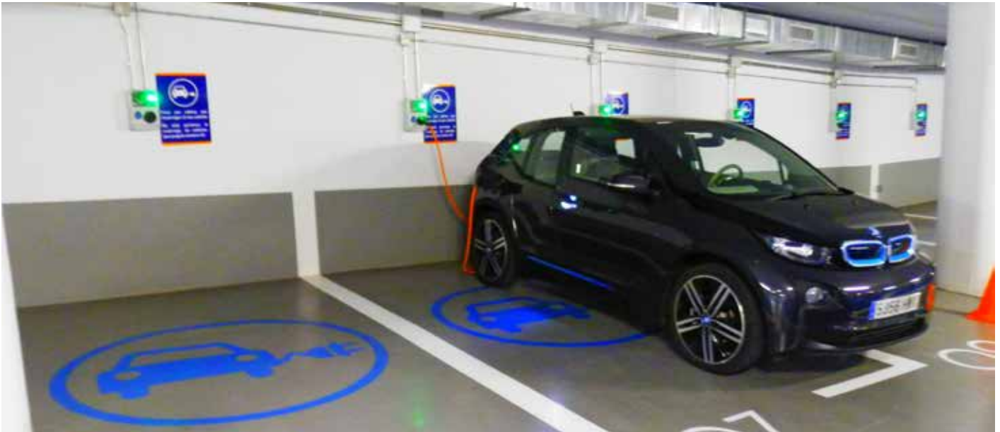
Newer apartment blocks are more likely to have EV charging bays, but older buildings may need electrical upgrades for this to be feasible.
