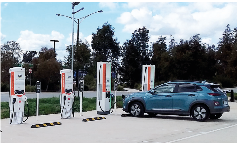
Charging at the Chargefox ultra-fast charger in Barnawartha North, in northern Victoria. There are two ultra-fast (350kW) chargers and two fast (50kW) chargers available.
