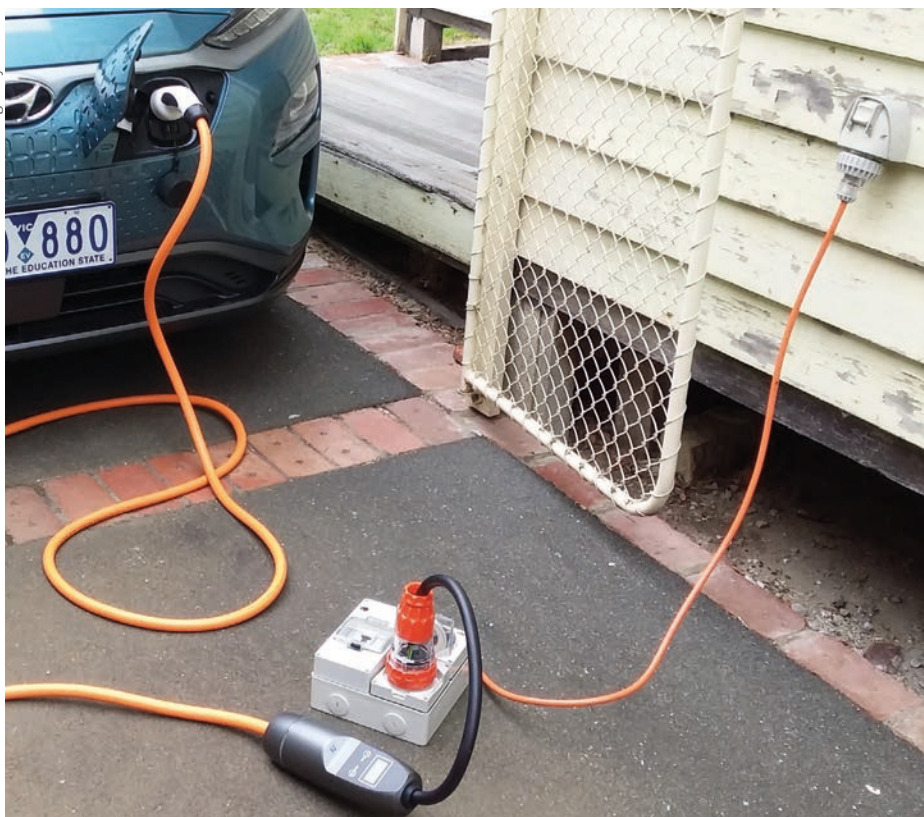
This Hyundai Kona is opportunity charging from a regular power point using a 22 kW, three-phase portable EVSE. To limit power draw to the power point's 10 A maximum, the EVSE must be set to 10 A or less. Note the impressive adaptor box which adapts the EVSE's five-pin (three-phase) plug to the 10 A power point. Most electricians should be able to make such adaptors. This one was assembled by Bryce Gatton, who can make them for customers on request.
